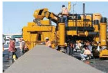
The wall has a 19 inch (483 mm) wide top, is 39.25 inches (997 mm) wide at the base and its sidewalls vary in height from 3.5 to 6.5 feet (1.1 to 2 m).
