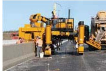
Stringline is set underneath the Commander III and out of the way of the finishers.
