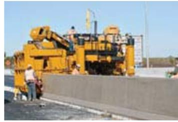
Slipforming successful wall, according to P.T. Ferro, is having the right concrete mix design delivered at the correct slump.
